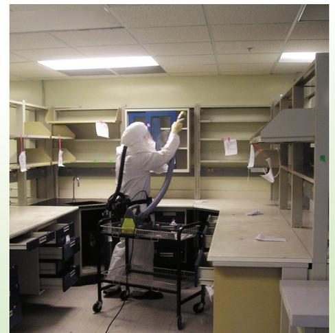
**A new facility was disinfected by treating with a liquid chlorine dioxide to provide a clean start for research taking place within the facility. A high concentration liquid chlorine dioxide was sprayed throughout the facility similar to a hydrogen peroxide vapor treatment. A team opened drawers, cabinets, and equipment in order to ensure that all visible surfaces were sprayed and treated with liquid chlorine dioxide. This method offers a level of disinfection comparable to utilizing VPHP.**
