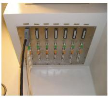
Tubing and wiring is run from distribution plate to the ceiling plate
